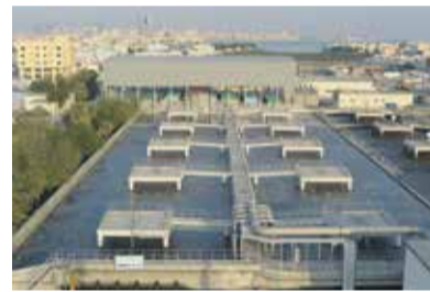
HYBACS installation at Tubli wastewater treatment plant, Bahrain
