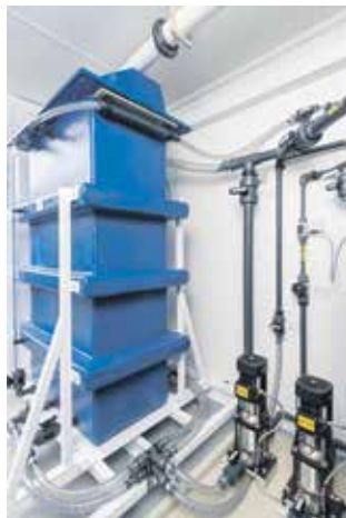
Nyex™ 7-100a reactor tank
