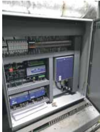
Open access control panels give AD operators full control over their own engine
