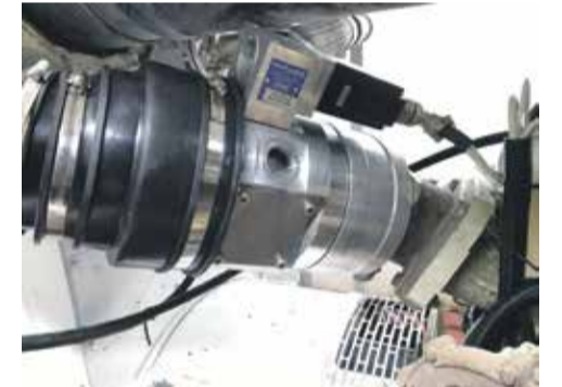
A flexible fuel mixer is essential for biogas plants treating sewage sludge
