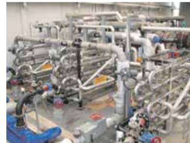
The HRS DTI Series of corrugated tube-in-tube heat exchangers is ideal for sludge applications
