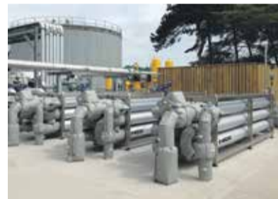
The HRS DTI Series has a proven record with difficult materials such as sludge and digestate
