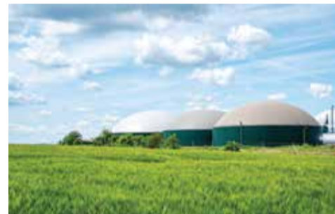
AD operators can improve their engine's performance with real-time CHP monitoring
