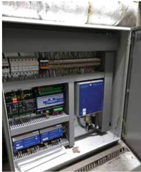
The Motortech open access control panel comes with the IGS-LOG as standard
