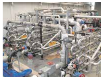
The HRS DTI Series of corrugated tube-in-tube heat exchangers is ideal for sludge applications
